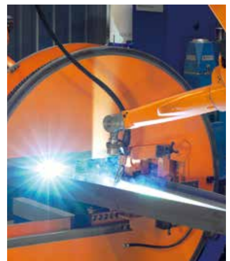
Robot plant to weld steel components for hall production.
